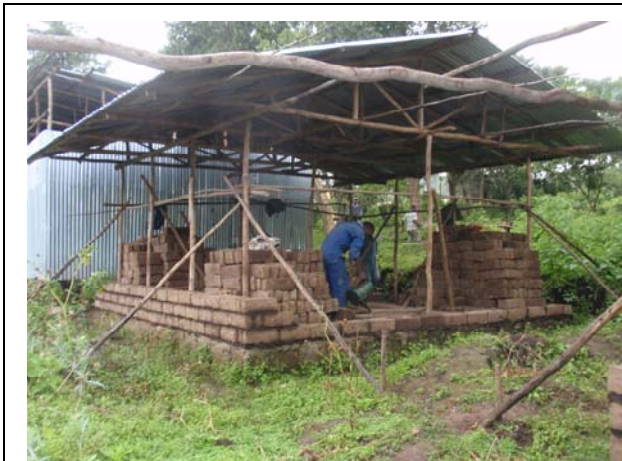
Murning under "temporärt tak"
